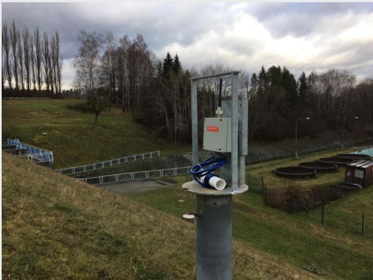
*Loadsensing data node installation at the Olešná Dam*
